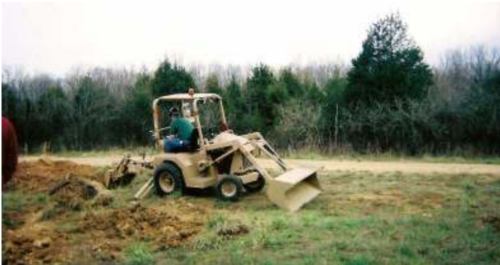
Machine searching in a culvert/drain pipe for IEDs
